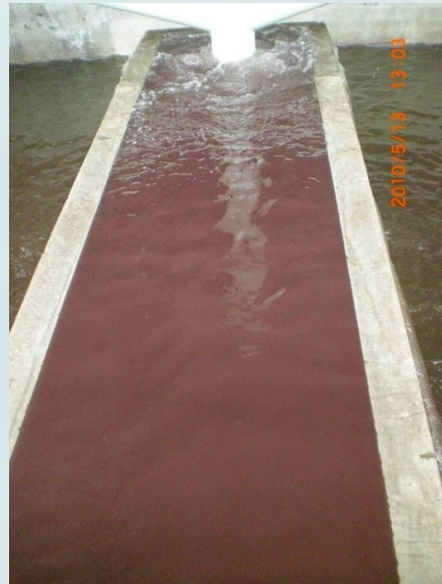
Waste Water Treatment View
