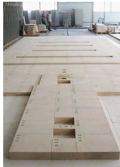
Melting tank bottom with big size light-weight insulation blocks
