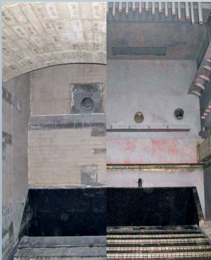
Stoker furnace steel housing with and without refractories
