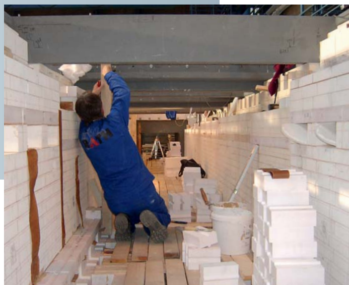
Assembly of a pusher-type furnace
