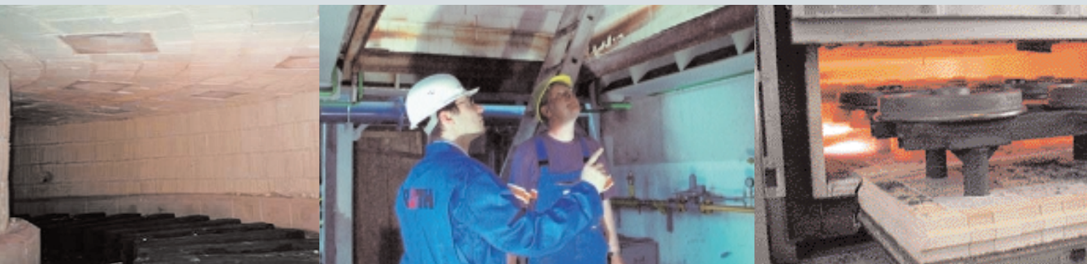
Rotary hearth furnace
