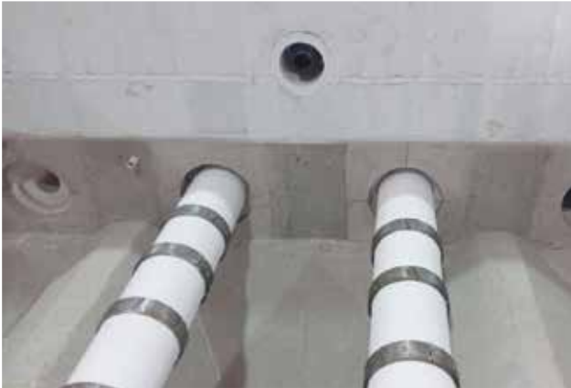
ALTRA roller insulation pre-assembled at the factory
