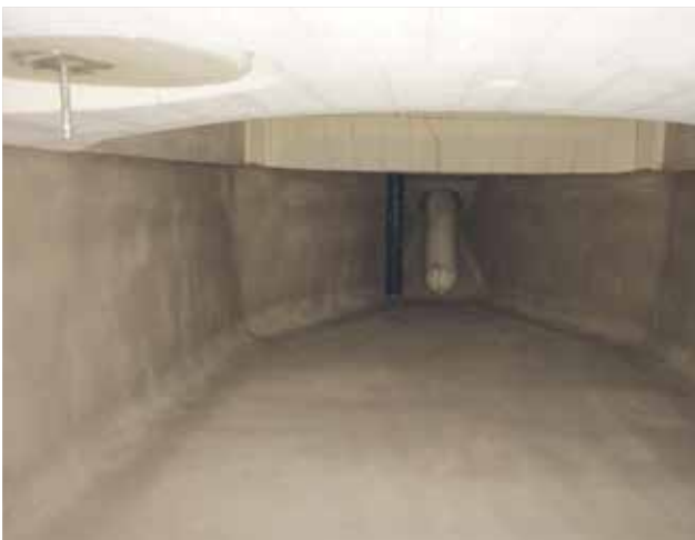
Dosing furnace–bath area with anodes
