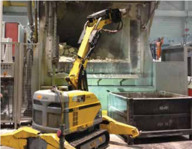
Chiseling out the old liner
