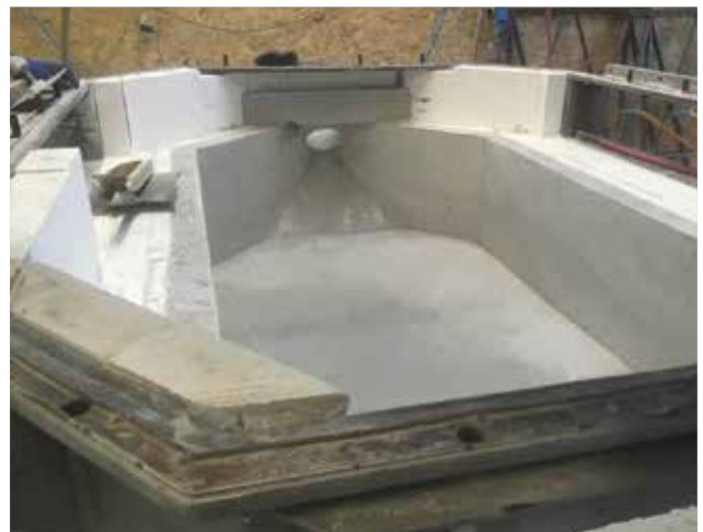
Dosing furnace–bath area
