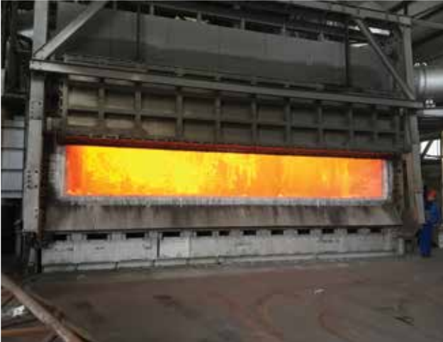
Single chamber smelting furnaces
