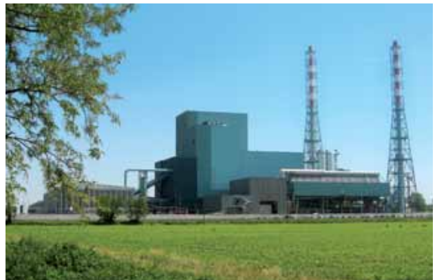
Incinerator - Courtesy of Lomellina Energia
